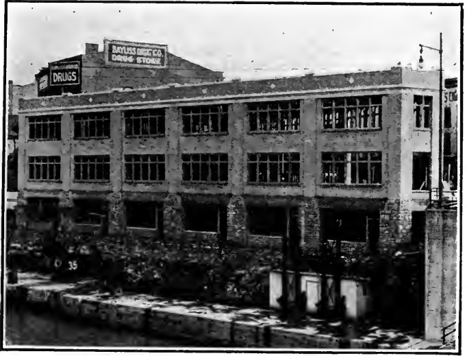
WHERE WAS FORMERLY A LOCAL EYESORE THE LOCKPORT, N. Y., BOARD HAS BUILT ITSELF AN ATTRACTIVE HOME
